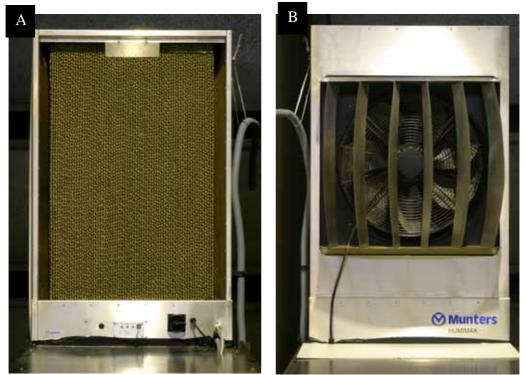
Munters HM2 4000 evaporative humidifier showing A) the evaporative media at the front (or intake side); and B) the fan blowing humidified air out into the store.
